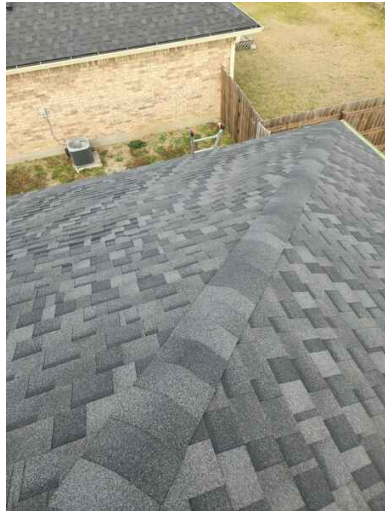
Types of Roof Covering: Asphalt Shingle Viewed From: Roof Surface Dimensional Asphalt Shingle Information:
