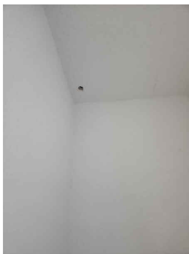
Closet of first bedroom on right
