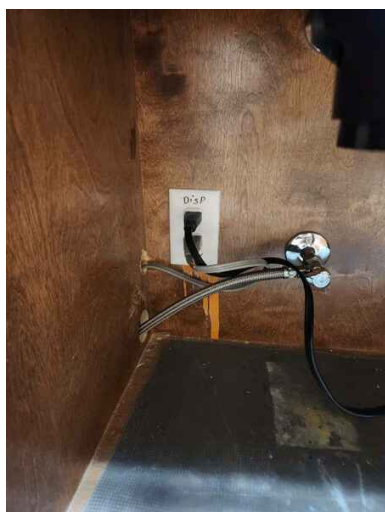
Dishwasher Plug in Under Sink
