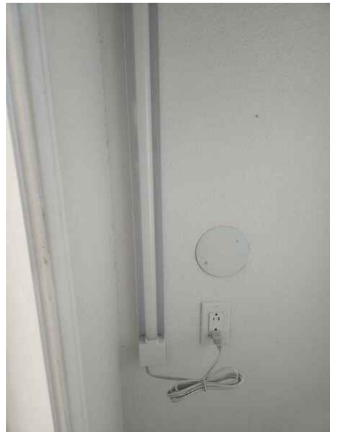
Front Bedroom Closet
