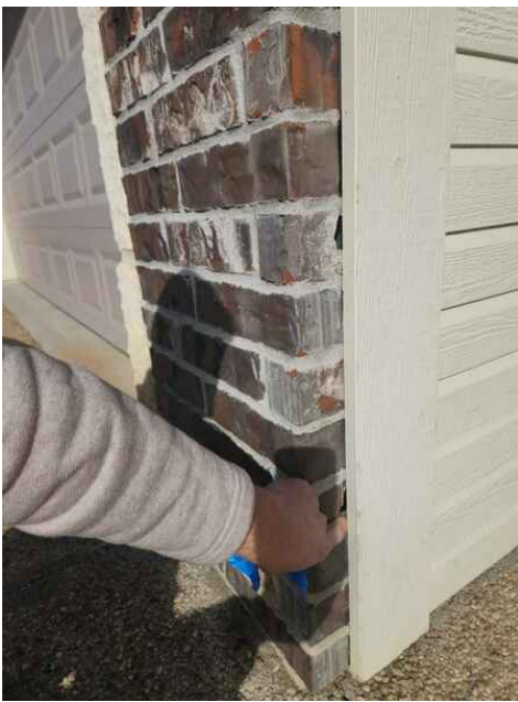
Front Entry Siding Transition
